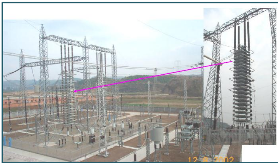
Figure (2.26): DC harmonic filter capacitors [29]
